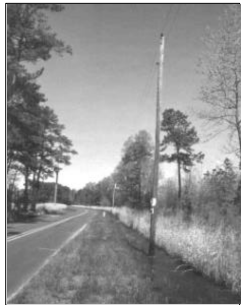
Figure 9. In some areas, properly treated poles, like the one above treated in 1947, spend most of their lives in water or water-logged soils. (Eastern shore of Maryland, United States)
