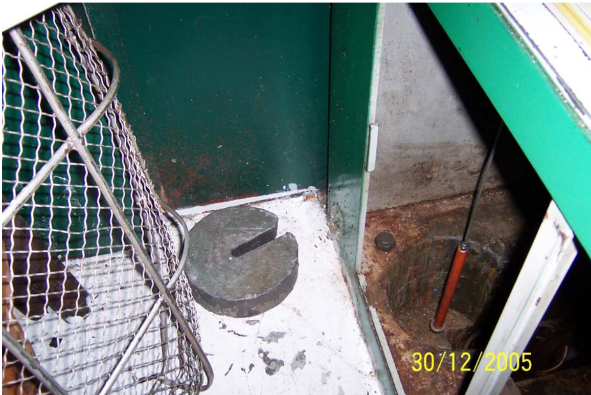
Figure 7: Logement des contrepoids
