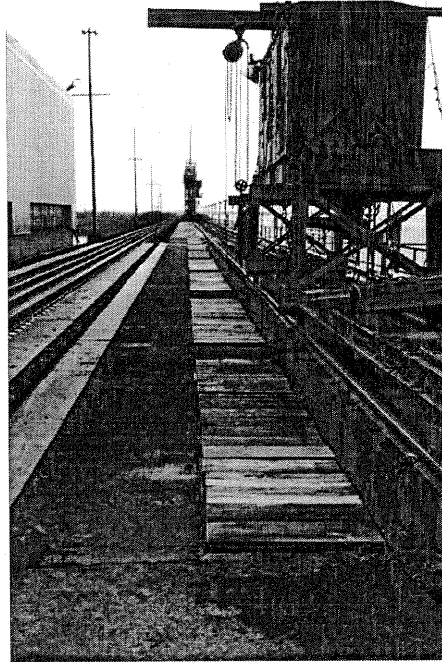
Photo 9: Chariot de manutention amont
