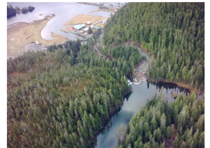
City of Pelican Hydroelectric Upgrade during construction Alaska Energy Authority
