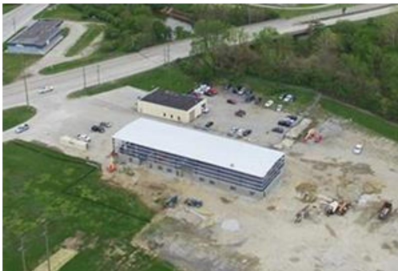
Southside LFG to RNG Plant Under Construction
