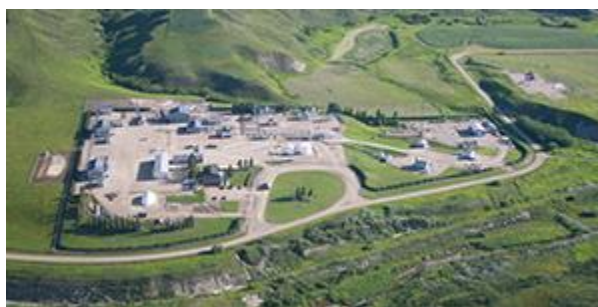
Natural gas storage facility, Carbon, Alberta
