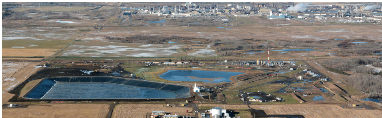
ATCO Heartland NGL storage facility, Fort Saskatchewan, Alberta
