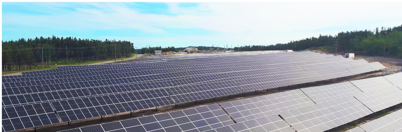
Fort Chipewyan Solar Project, Fort Chipewyan, Alberta
