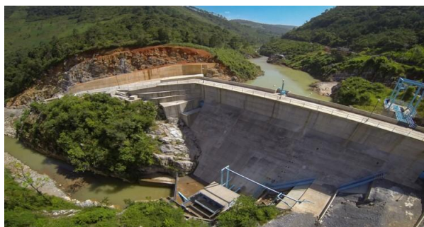
Hydroelectric power station, Veracruz, Mexico
