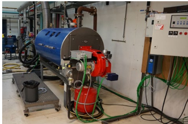
Figure 6-28: 475 kw boiler equipped with a 475 kW forced-draught burner [64]
